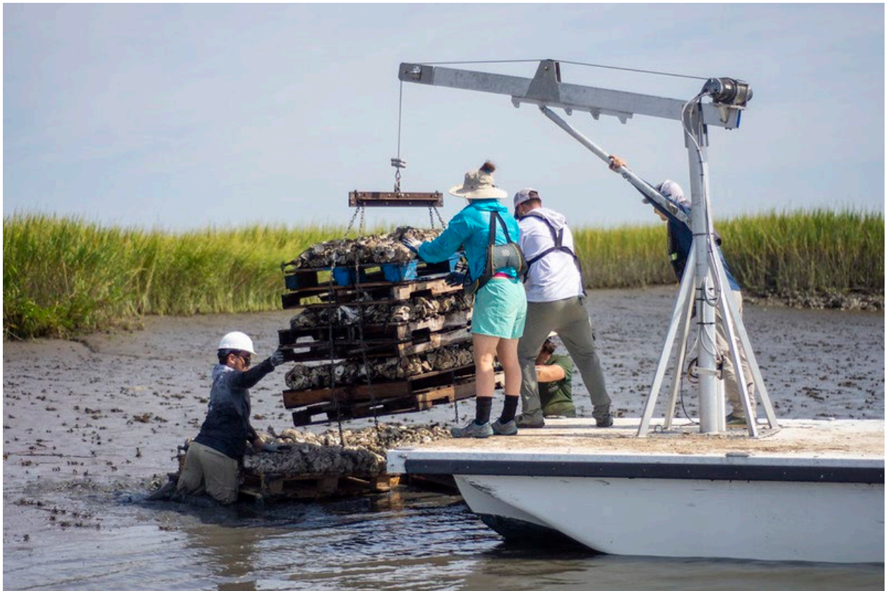
Bagged oyster shells from shell recycling program being deployed via wooden pallets onto the bank of the North Newport River, Georgia as part of an oyster restoration project. Credit: Tyler Jones (GADNR)
