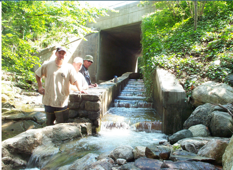
Furnace Brook Fishway. Photo (c) CT DEEP
