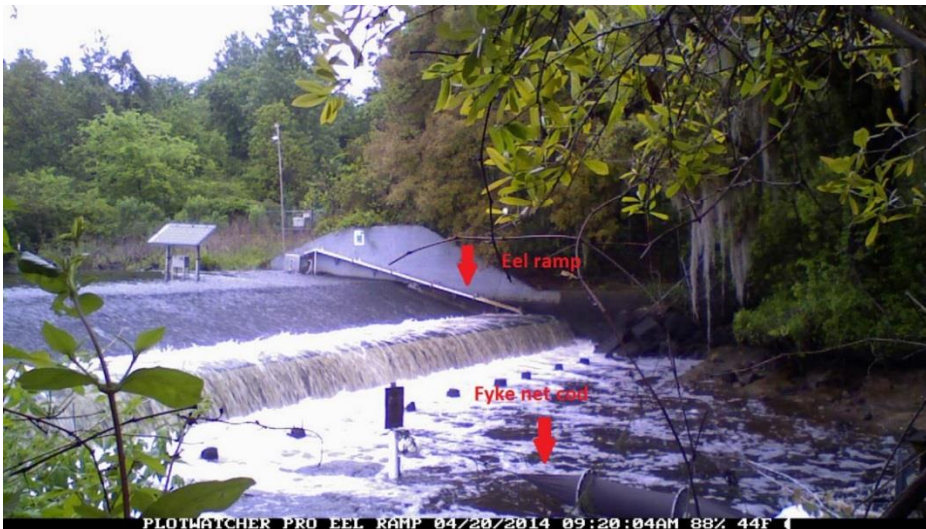
Figure 10. Goose Creek Reservoir spillway and red arrows indicating the locations of the fyke net and eel ramp.
