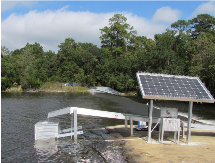
Figure 9. Solar power eel ramps (2) located adjacent to the spillway of Goose Creek Reservoir, South Carolina.
