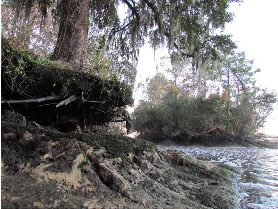
Figure 8. Bank erosion has washed away nearly all of the soil from underneath the tree making it susceptible to falling into the sampling area.
