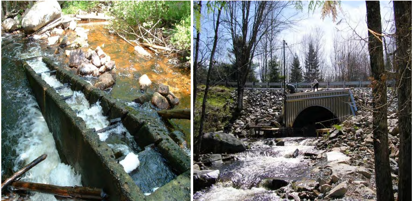
Fishway leading to spawning habitat in Flanders Pond prior to fall of 2012 (left). Removal of the fish ladder and installation of a bottomless arch culvert ready for the 2013 alewife migration (right).
