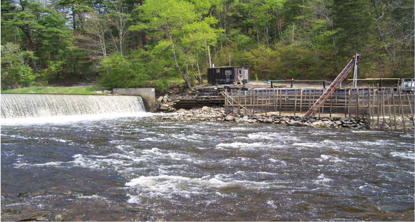
Tidal weir located in Orland, Maine
