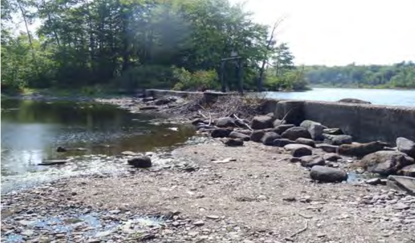
Existing outlet dam at Pushaw Lake prior to fishway installation
