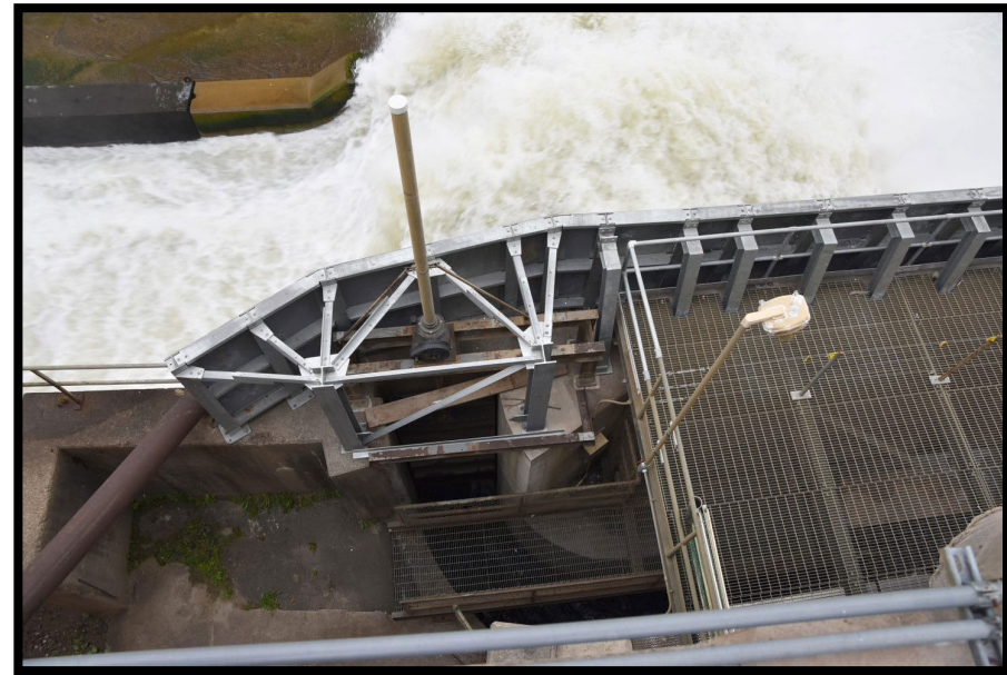
Fish elevator entrance at Holyoke Dam, Holyoke, CT. Credit: A. Miehl.
