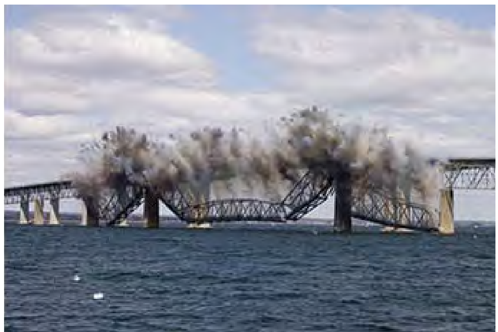
Figure 11. The through truss span of the Old Jamestown Bridge, just before it hits the water following the first controlled explosive demolition in 2006. Photo credit: RIDOT.
