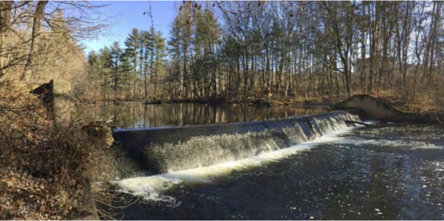
Dana Dam (Wilton, CT)
