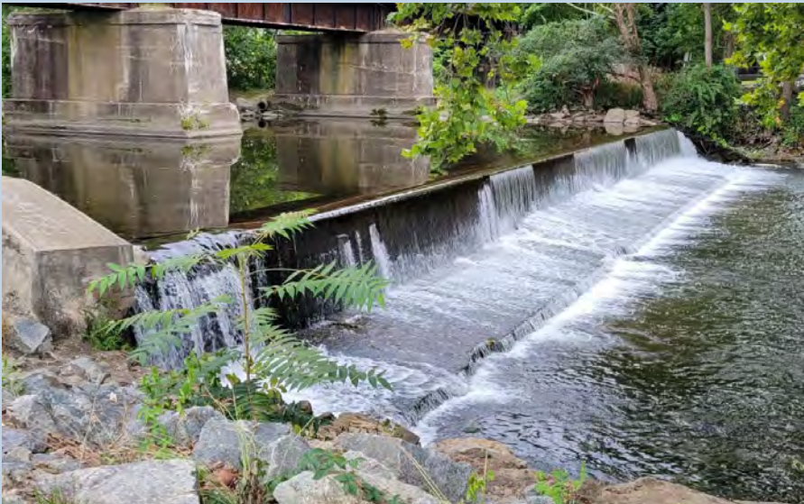
Lower E.R. Collins Dam - funded in FY23
