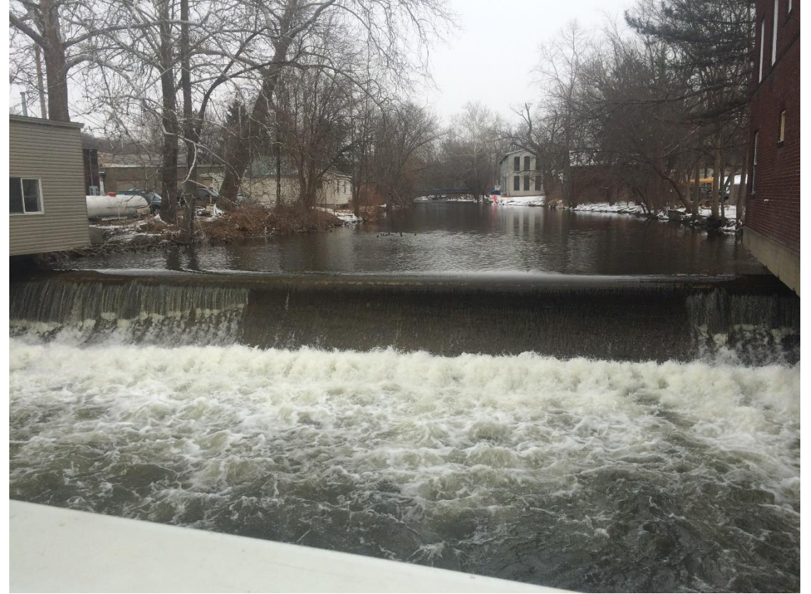
Upper E.R. Collins Dam
