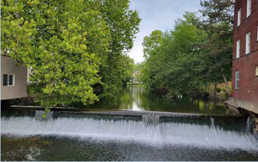
Upper E.R. Collins Dam (credit: TNC)
