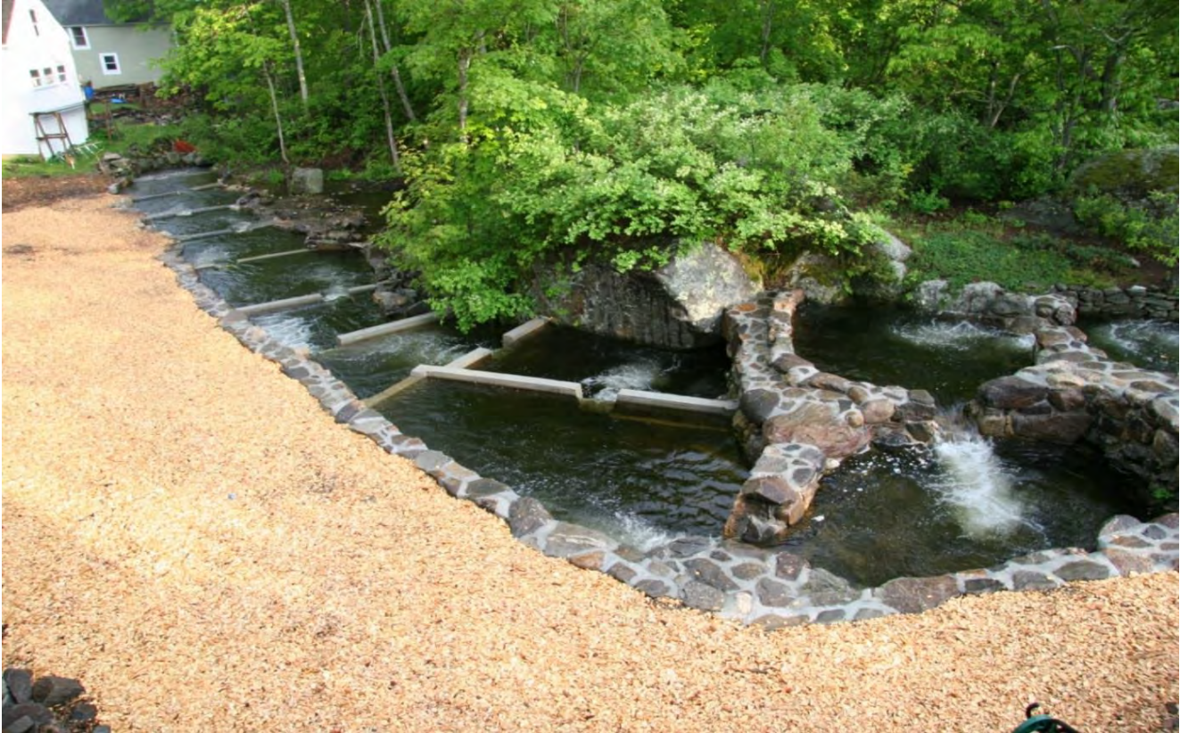
Upper section of the fishway after restoration.
