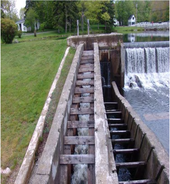
Tidal Denil fishway located in Some Harbor and Some Brook leading to Some Pond.
