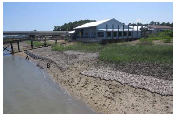
South Carolina DNR deploys (A) oyster castles, (B) concrete-coated crab traps, and (C) bagged shell as living shorelines. Photo credit: SC DNR.
