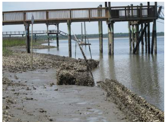
1 year after living shoreline installation. Photo credit: SC DNR.
