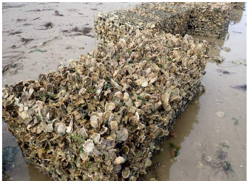
Dense oyster growth on MWRs at Fort Johnson approximately 11 months after installation. The rapid recruitment of oysters to the wire structures demonstrates how quickly living shorelines can become established in the environment and provide essential fish habitat as well as shoreline protection. Image credit: SCDNR.
