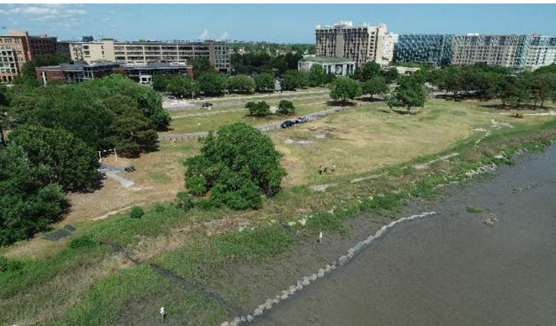
Wire-based living shoreline at Brittlebank Park in downtown Charleston. Other living shorelines at Brittlebank Park have demonstrated successful marsh grass recruitment and sediment accumulation which provides shoreline protection and wave attenuation. Image credit: SCDNR.
