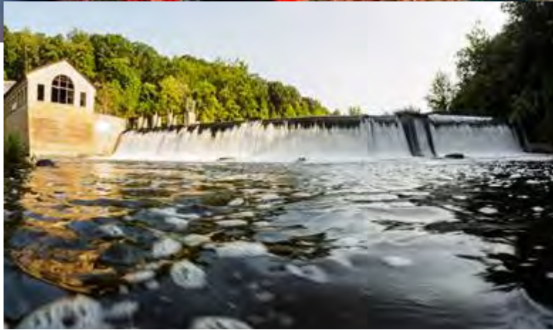
The Columbia Lake Dam removal is a $7 million project in Knowlton Township, NJ. Photo credit: NJDEP.
