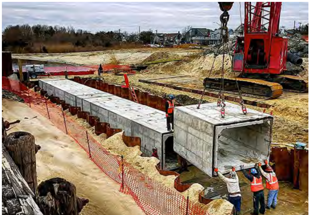
Working on the Wreck Pond Inlet Project. Photo credit: NJDEP.
