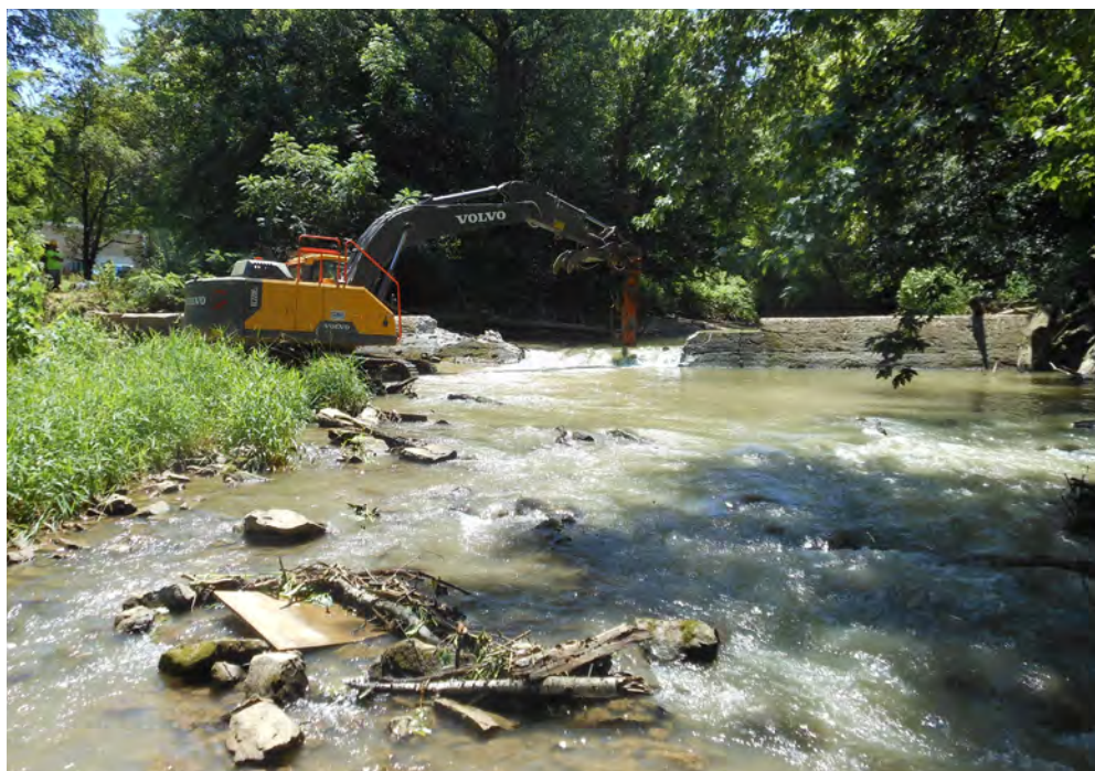
The removal of Krady Mill Dam, Chiques Creek, Lancaster County, PA. Photo credit: PFBC.
