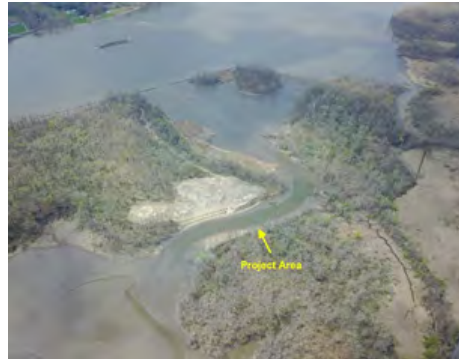
Project area post-construction, NYS Statewide Digital Orthoimagery. Photo credit: A. Hendry, McGill University.
