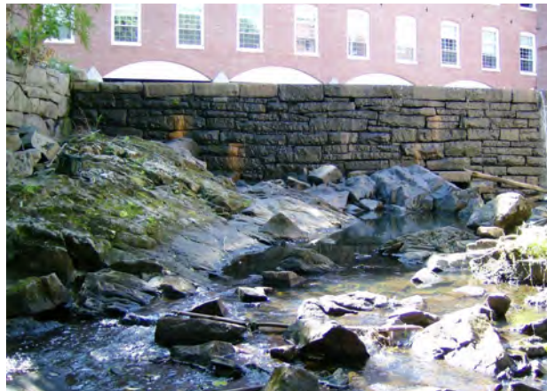
Lower Sawyer Mill Dam, which is scheduled to be removed in 2018. Photo credit: K. Lucey.
