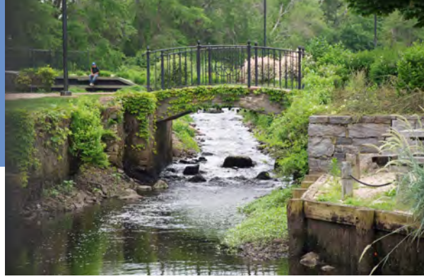
Grangebel Park rock ramp/nature-like fishway on the Peconic River in Riverhead, NY, completed in 2010. Photo credit: Peconic Estuary Program.
