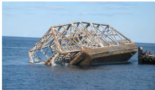
The 168-foot truss of the Highway 41 swing bridge, welded to the deck of a barge, being deployed on the Charleston Deep Reef MPA (left). Photo credit: SCDNR. The 106-foot tug, General Oglethorpe, being deployed on Comanche Reef (right). Photo credit: SCDNR.
