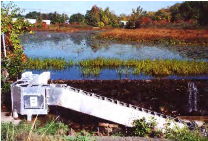
The fishway with viewing window at the Lilly Pond Dam, a 5-foot high dam originally built in 1790.
