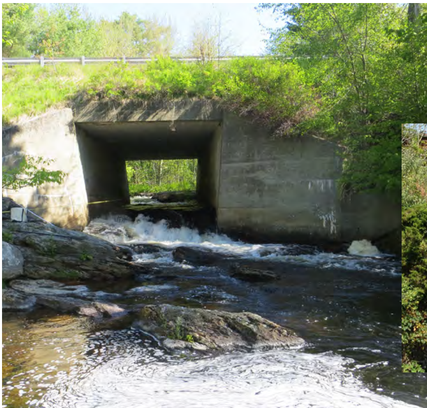
Nature-like rock weirs will replace the temporary fish ladder at the Route 172 crossing on Patten Stream to allow for fish passage. (Source: Town of Surry)
