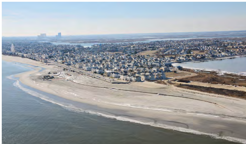
New Jersey Shore Protection: Brigantine Inlet to Great Egg Harbor. (Source: US Army Corps of Engineers)
