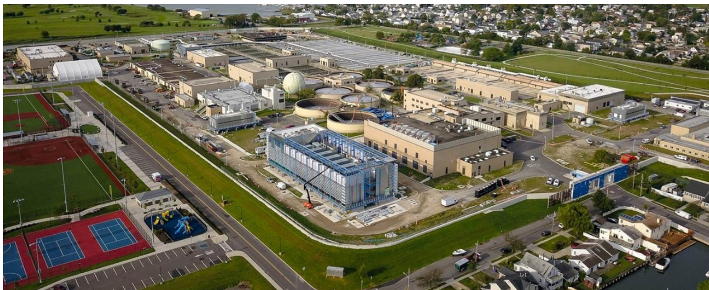
Aerial view of the South Shore Water Reclamation Facility, Nassau County, NY. Photo credit: Veolia North America
