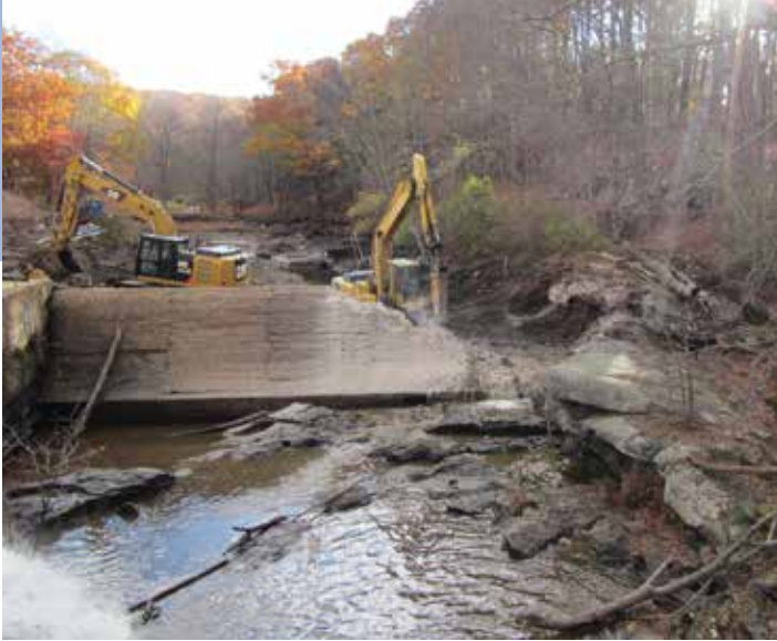
Early Breach- The Norton Mill Dam Removal on the Jeremy River opened 17 miles of diadromous fish habitat. Photo credit: CTDEEP
