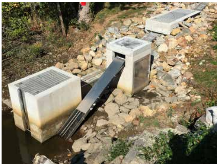
Chapmans Pond Dam is at the head-of-tide on the Menunketesuck River. The steeppass fishway on the left passes river herring; the eel pass on the right collects eels that drop into a trap where they are enumerated and carried around the dam. The substrate to the left is for glass eels; the substrate on the right is for larger yellow eels. Photo credit: CT DEEP
