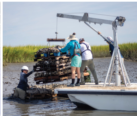
Left: Volunteers build gabions filled with oyster shell as part of an upcoming project projected to be the largest oyster restoration in Georgia’s history in Teakettle Creek. Right: Staff of the Georgia Department of Natural Resources Coastal Resources Division and volunteer students from Georgia Southern University restore the bank of the North Newport River as part of a carbon sequestration study. Photo (c) Georgia Department of Natural Resources.
