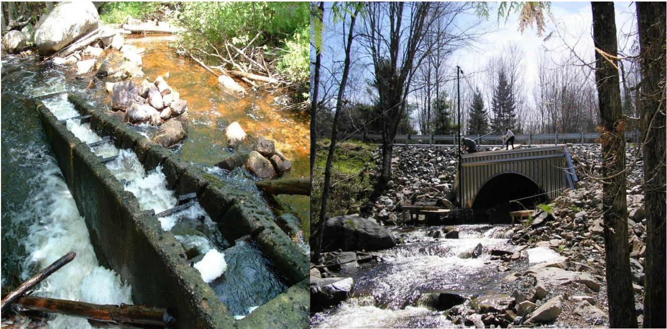
Figure 25. Fishway leading to spawning habitat in Flanders Pond prior to fall of 2012 (left). Removal of the fish ladder and installation of a bottomless arch culvert ready for the 2013 alewife migration (right).
