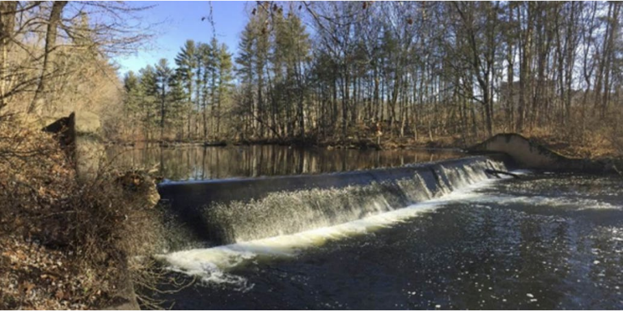
Dana Dam (Wilton, CT)
