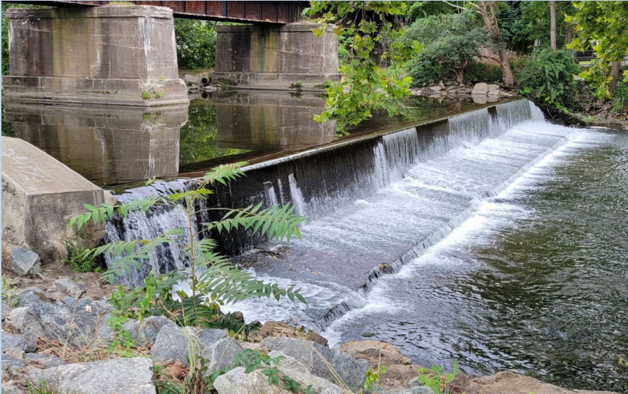
Lower E.R. Collins Dam - funded in FY23
