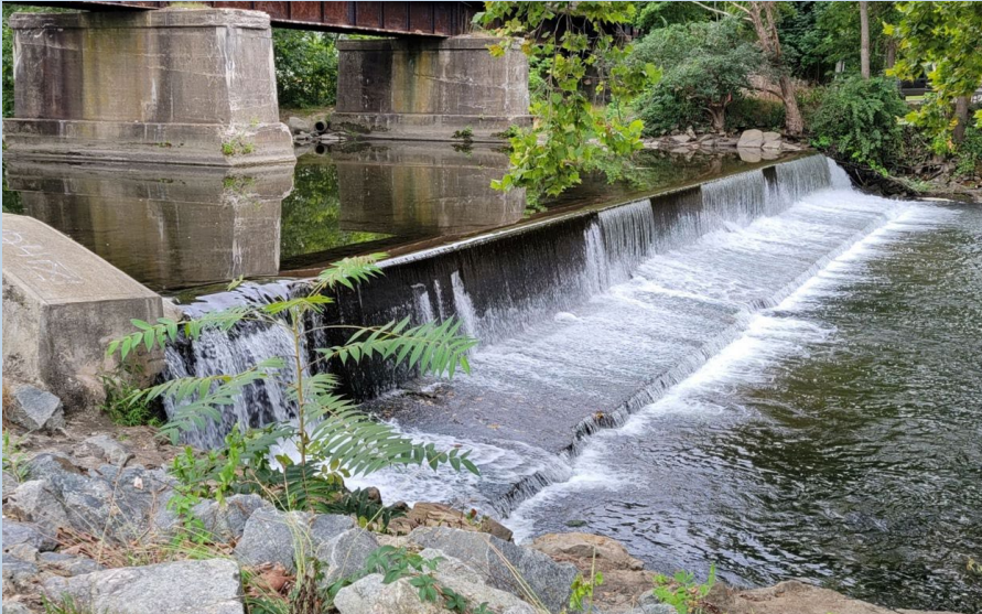
Lower E.R. Collins Dam - funded in FY23
