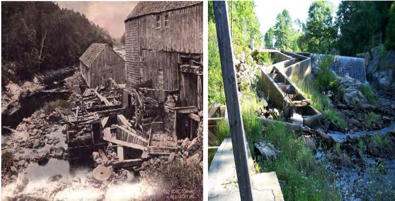
Historic picture of the Nequasset Mill and fish passage to spawning habitat and the trapping facility prior to 2014 rebuild.
