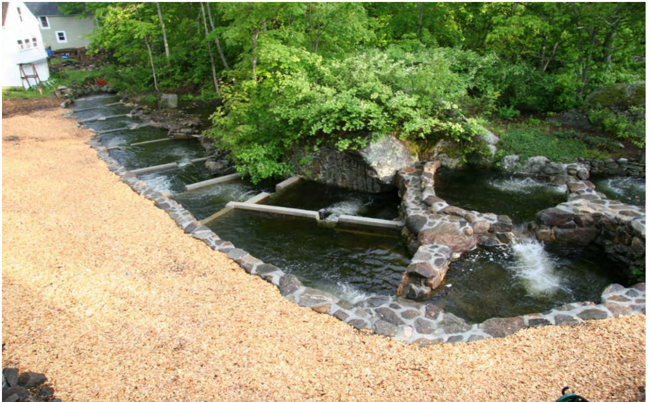
Upper section of the fishway after restoration.
