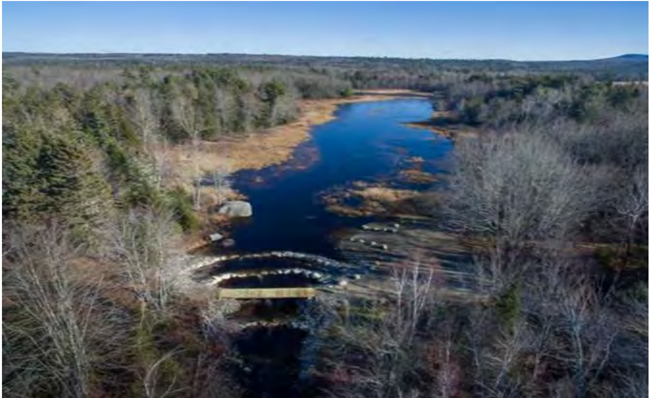
Nature-like fishway installed at Wights Pond
