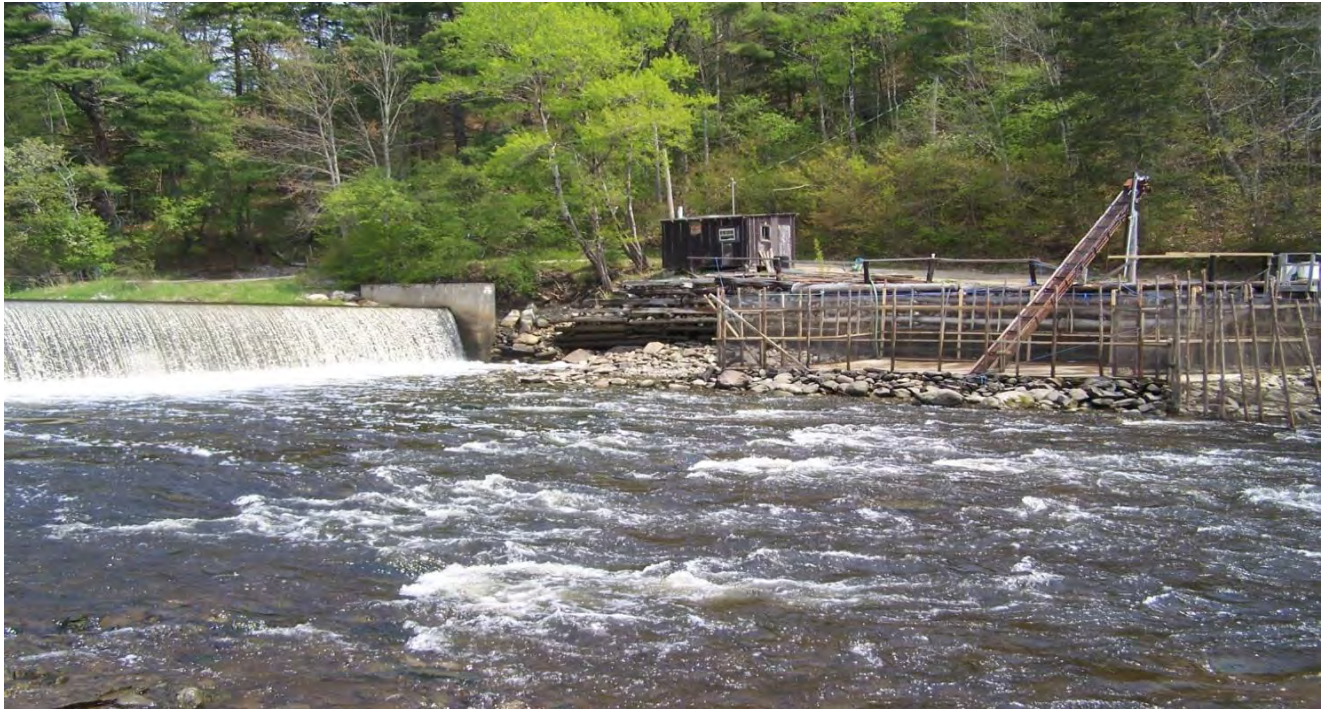
Tidal weir located in Orland, Maine
