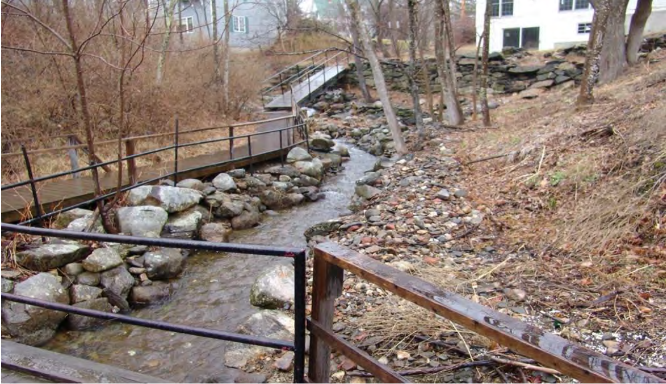
Entrance to the Damariscotta fishway.
