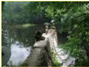
Sennebec Lake Dam, ME
