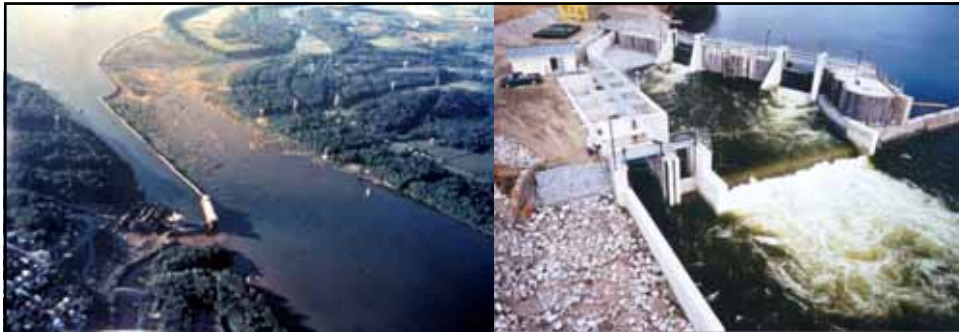
York Haven Dam and Fishway
