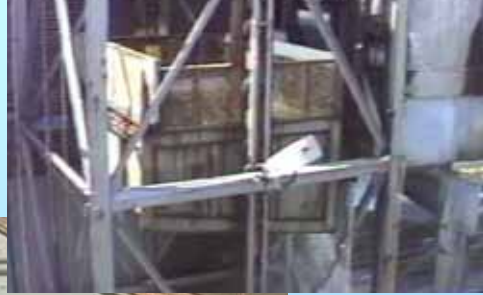
Holyoke fish lift, Holyoke Dam, Connecticut River, MA
