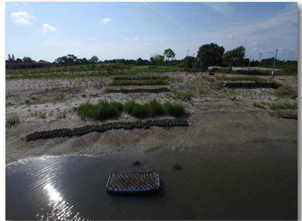
The Shoreline Demonstration Area (from left to right): native plants, native plants with oyster bags, terracing with oyster bags, a kayak launch, a retaining wall with oyster bags. Photo credit: http://floridalivingshorelines.com/ .
