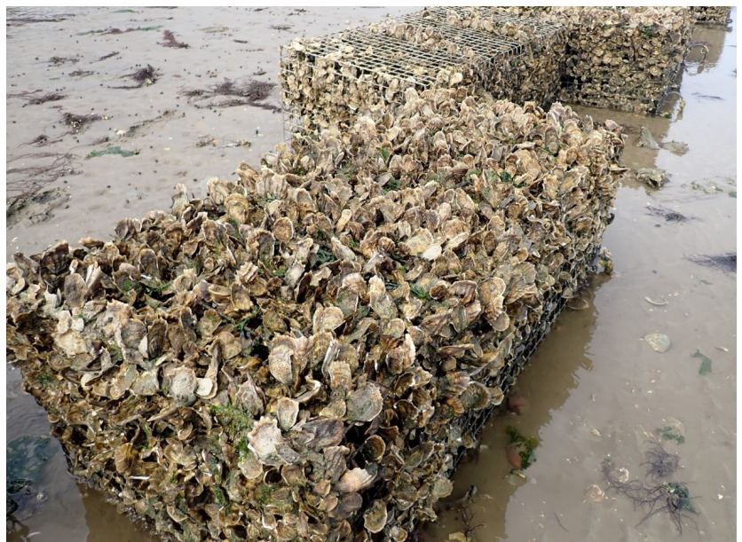
Dense oyster growth on MWRs at Fort Johnson approximately 11 months after installation. The rapid recruitment of oysters to the wire structures demonstrates how quickly living shorelines can become established in the environment and provide essential fish habitat as well as shoreline protection. Image credit: SCDNR.
